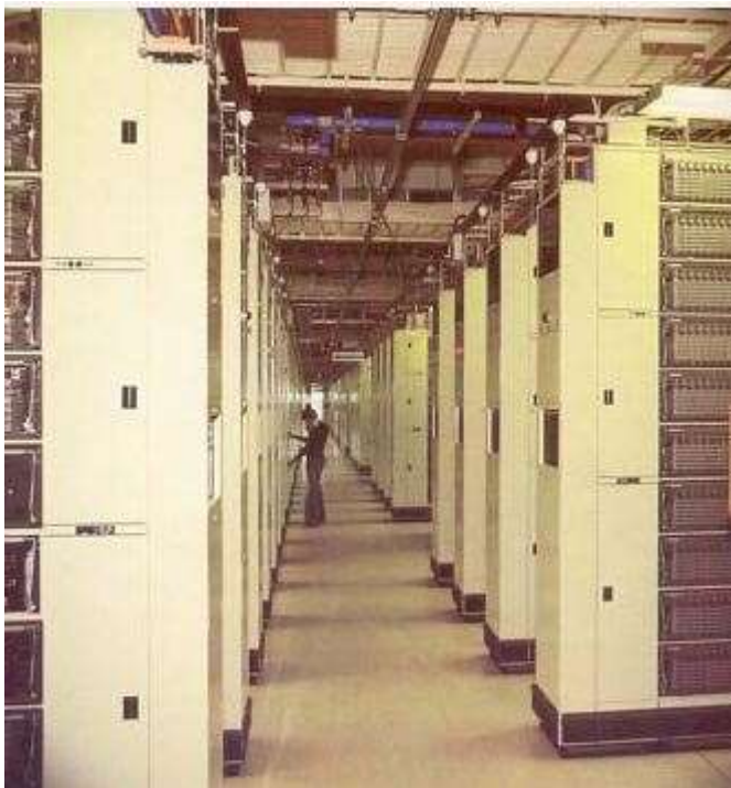
Figure 18—Mondial 1, general view of TXK2
